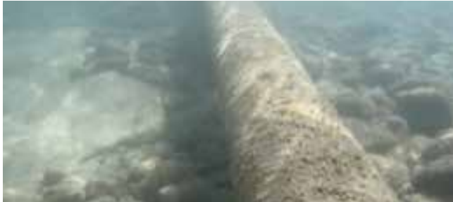
Figure 7. Underwater image of the pipeline (Source: author).
